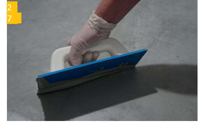
The covering is grouted after the covering surface is ready to be walked on. Due to the lack of absorbency of plastic mats, the curing time of the adhesive must be expected to be 3 to 4 times longer than for absorbent substrates.
