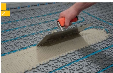
The sealing adhesive is applied to the joint areas of IndorTec® THERM-E or to the connection areas of adjacent components in accordance with the manufacturer's instructions.
