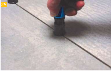
IndorTec® FN leveling aids can be used to prevent overtoothing at the top of the pavement.
