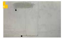
Insert the IndorTec® THERM-E TD temperature sensor into the recess provided, run the supply cable into the switch box and fill the recess in the supply cable with adhesive mortar. The position of the heating foil, the supply lines and the temperature sensor must be documented in the installation plan.
