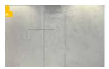
Wall surfaces to which the IndorTec® THERM-C wall heating is to be attached must be marked before installation. The same applies to the recesses for supply lines, the contacting of the heating foil, the IndorTec® THERM-C wall heating and the IndorTec® THERM-E TD temperature sensor. The processing guidelines for the temperature sensor must be observed.
