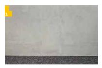
Prepare a level, clean, load-bearing substrate. Drywall boards and wood-based panels must be crack-bridging in the joint area. The IndorTec® THERM-E thermal barrier can be used to improve heat radiation and additionally bridge cracks in the substrate.
