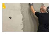
Once the adhesive mortar has dried through, the IndorTec® THERM-C wall heating can then be fully covered with a minimum 2 mm thick top layer of filler, a plaster system ...
