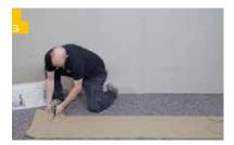
After the resistance test of the heating foil, the IndorTec® THERM-C wall heating, it can be individually processed and cut to size according to the installation guidelines.
