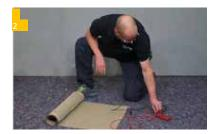
Before installing the heating foil, the IndorTec® THERM-C wall heating and the IndorTec® THERM-E temperature sensor, the total resistance must be checked and recorded in accordance with the acceptance protocol. The heating foil of the IndorTec® THERM-C wall heating system must not have been processed or shortened.
