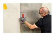
Then cover the entire surface of the heating foil of the IndorTec® THERM-C wall heating system with a layer of adhesive mortar and smooth it down.
