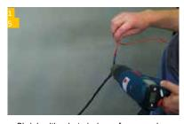
z. Shrink with a hot air dryer, for example. Pay attention to the maximum permissible length of the supply cable. To be on the safe side, we recommend carrying out another check resistance test on the heating foil of the IndorTec® THERM-C wall heating.
