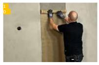
...insert the heating foil of the IndorTec® THERM-C wall heating into the adhesive mortar layer and align, the visible copper strip must be laid towards the wall. When using several heating foils of the IndorTec® THERM-C wall heating, keep a distance of at least 2 cm between the foils.
