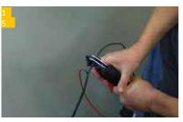
The connection cable of the heating foil, the IndorTec® THERM-C wall heater, is connected to the safety transformer (power supply unit). To do this, crimp the connection cable of the heating foil, the IndorTec® THERM-C wall heating, firmly to the twin cable with the enclosed shrink connectors using crimping pliers and
