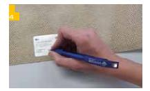
After processing or cutting, the resistance of the heating foil, the IndorTec® THERM-C wall heating, must be checked again and recorded on the product label and in the acceptance report.
