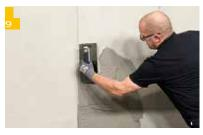
Apply the adhesive mortar to the marked surface using a suitable notched trowel (e.g. 4 mm notched trowel for a smooth substrate) to match the substrate, ...
