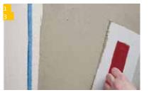
Heating foils from IndorTec® THERM-C wall heating must not be laid over expansion joints. A distance to the movement joint of min.
