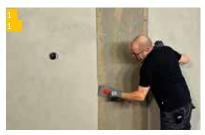
Press the heating foil of the IndorTec® THERM-C wall heating into the adhesive mortar layer using a plastic smoothing trowel, avoiding creases and folds in the foil at all costs.
